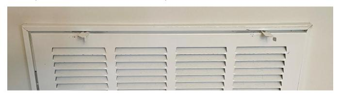
Once the tabs have been opened, the door over the filter can be pulled out and down, as shown above.
