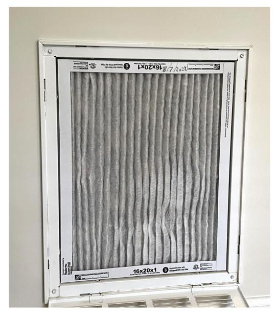
The standard 16" X 20" X 1" filter can be pulled out and replaced. New filters can be purchased at:
