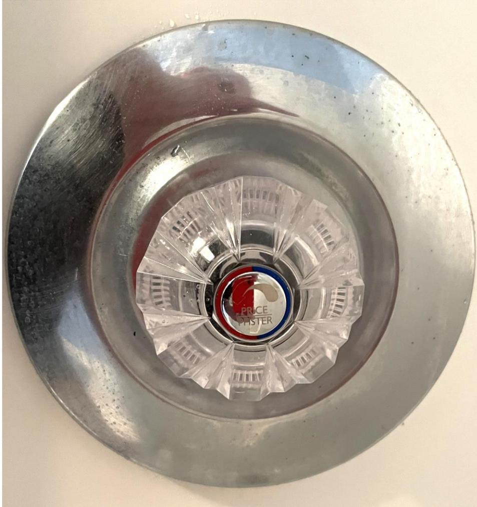
The center cap can be removed with a finger nail. Under this cap is a Phillips head screw which must be removed in order to take off the shower handle.
