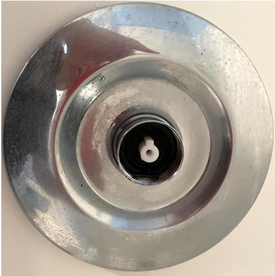
Once the handle is removed you will see the valve cartridge, a threaded collar and the faceplate. Remember the orientation of the center post – the protrusion will be pointing **UP!**
