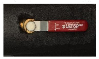
NOTE: The indications on the valve are NOT always correct. In the photo above, the handle indicates that the valve should be in a vertical position to be open. That is not how this installation works – the valve is installed backwards.
