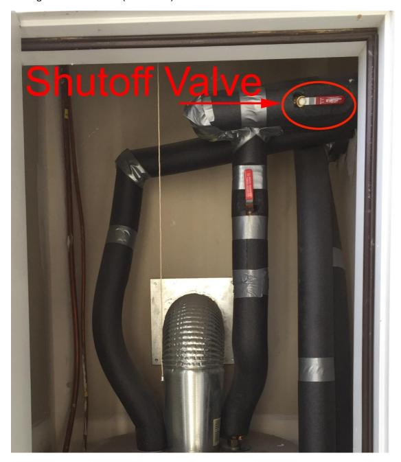
The valve shown above is closed by moving the red handle  $90^{\circ}$  to a vertical ( $\uparrow$ ) position.
